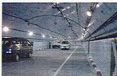
Đường ngầm 2 tầng Kuala Lumpur 9km flood tunnel - 3km road tunnel
